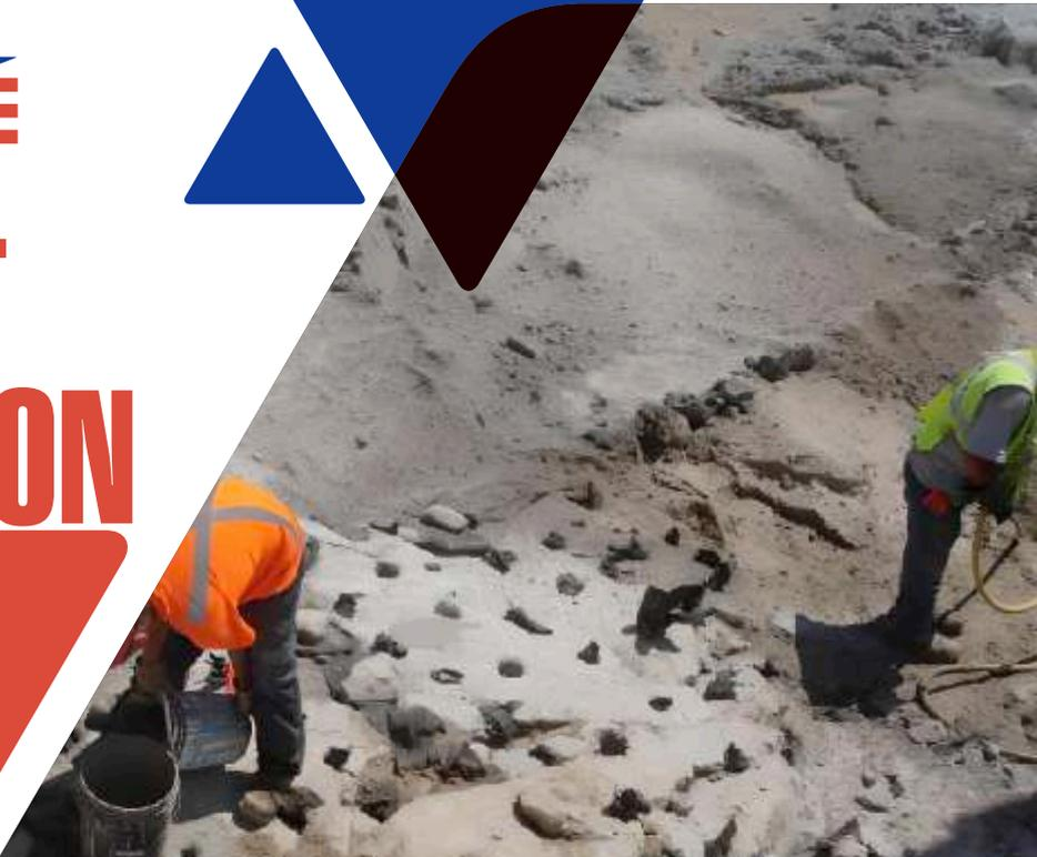
**CRACKAMITE is a non-explosive controlled demolition agent which works by providing silent expansive cracking for rock breaking, stone quarrying, mining, concrete demolition, excavation and more...**
