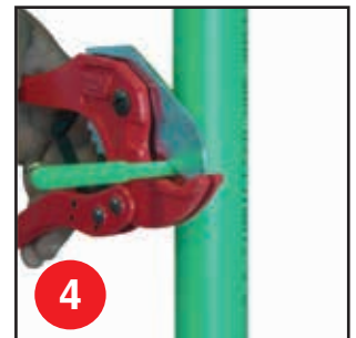
After cooling, cut the repair bar projected outside the pipe line using pipe cutter.
