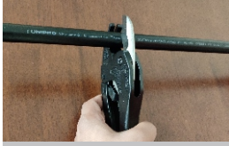
Step 1: Cut Unipro Metco Pipe at 90° angle
