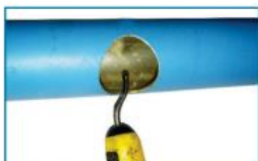
Step 4: Chamfering the hole
