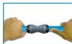
Step 3: Inserting the tubes into fitting
