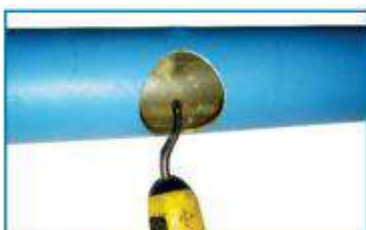
Step 4: Chamfering the hole
