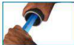
Step 2: Chamfering the Tubes
