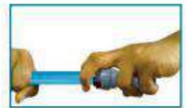
Step 4: Inserting the Tubes into fitting
