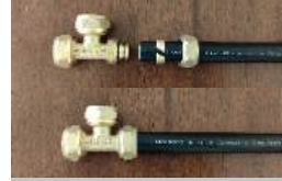
Step 4: Insert fitting and tighten nut with spanner to complete jointing.
