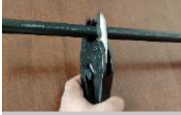
Step 1: Cut Unipro Metco Pipe at 90° angle
